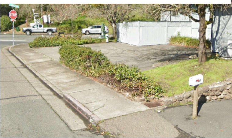
CONDITION 43 & 45 replace section of driveway apron w/ Sidewalk. Install sidewalk warp behind driveway apron
