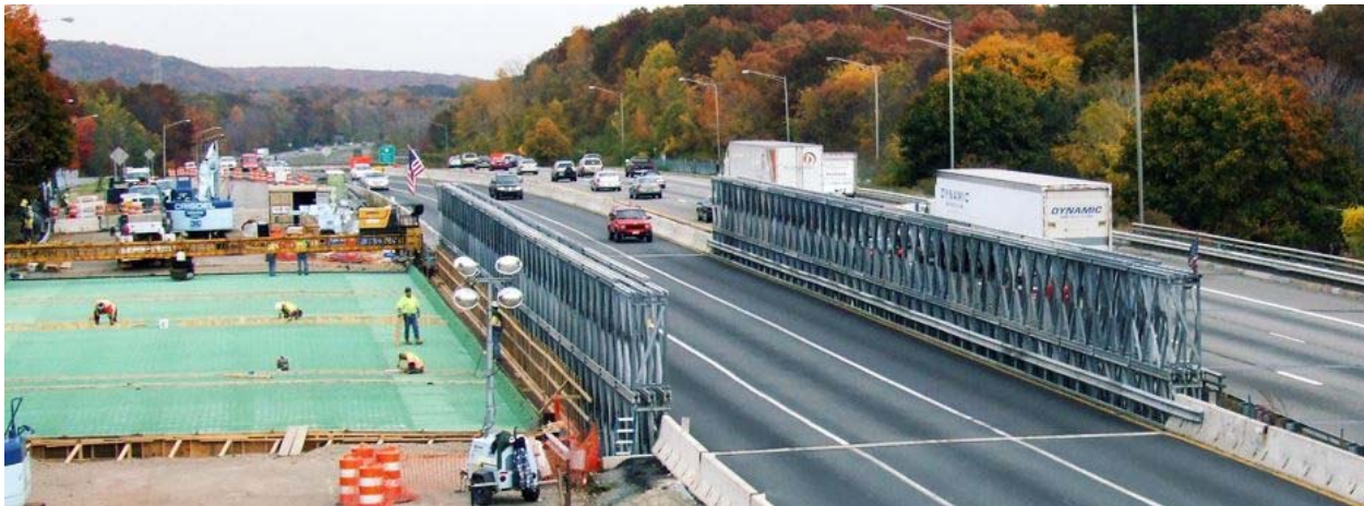
Figure 1 – ACROW Bridge used to Maintain Vehicular Traffic during Construction
