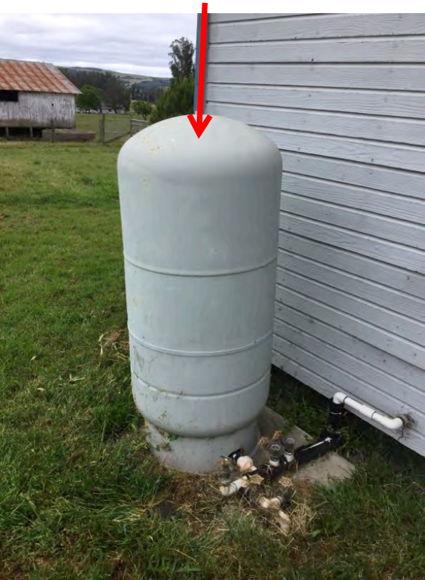
119 Gallon Pressure Tank (Behind Second Unit)
