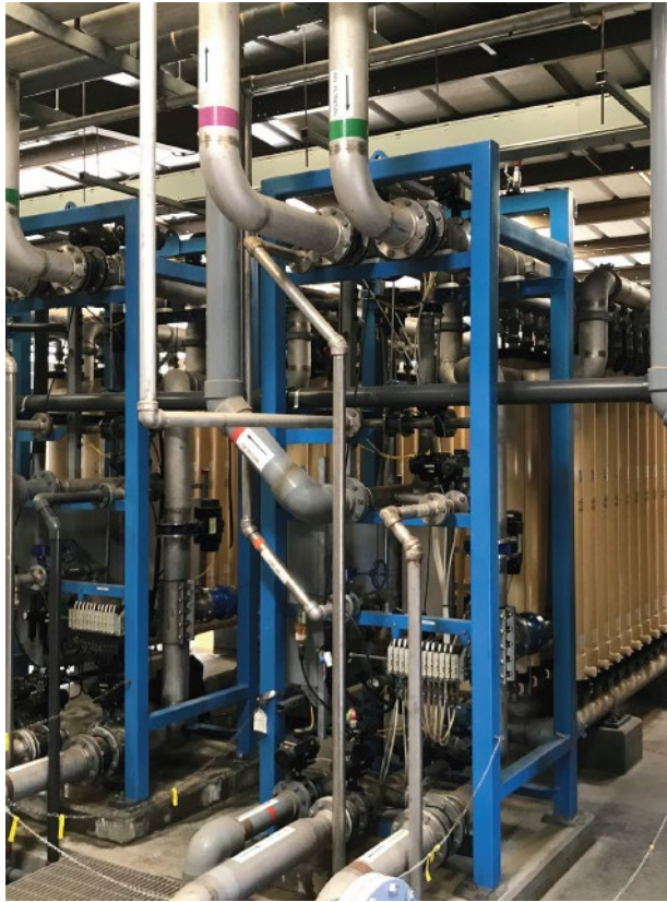
Airport: Microbe membrane filtering system modifications
