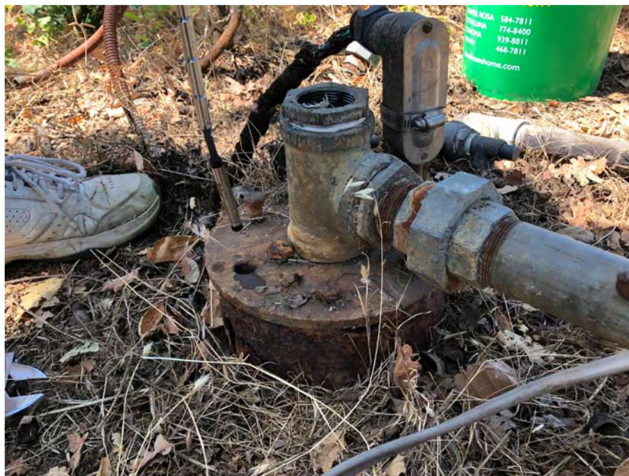
Figure 2 Monitoring well flange and reference point (see wet area at edge of access hole).
