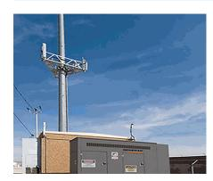
FIRE RESILIENCY and RECOVERY PROGRAM: Project will fund backup generators for installation at County maintained public safety communication sites. Backup generators are crucial to ensuring continuity of public safety radio communications during natural disasters and PG&E Safety Power Shutdowns.
