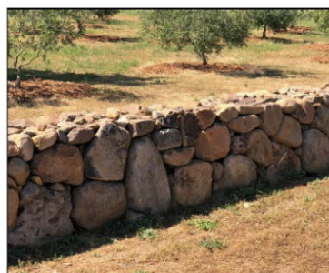
DRY STACK LOCAL STONE WALLS
