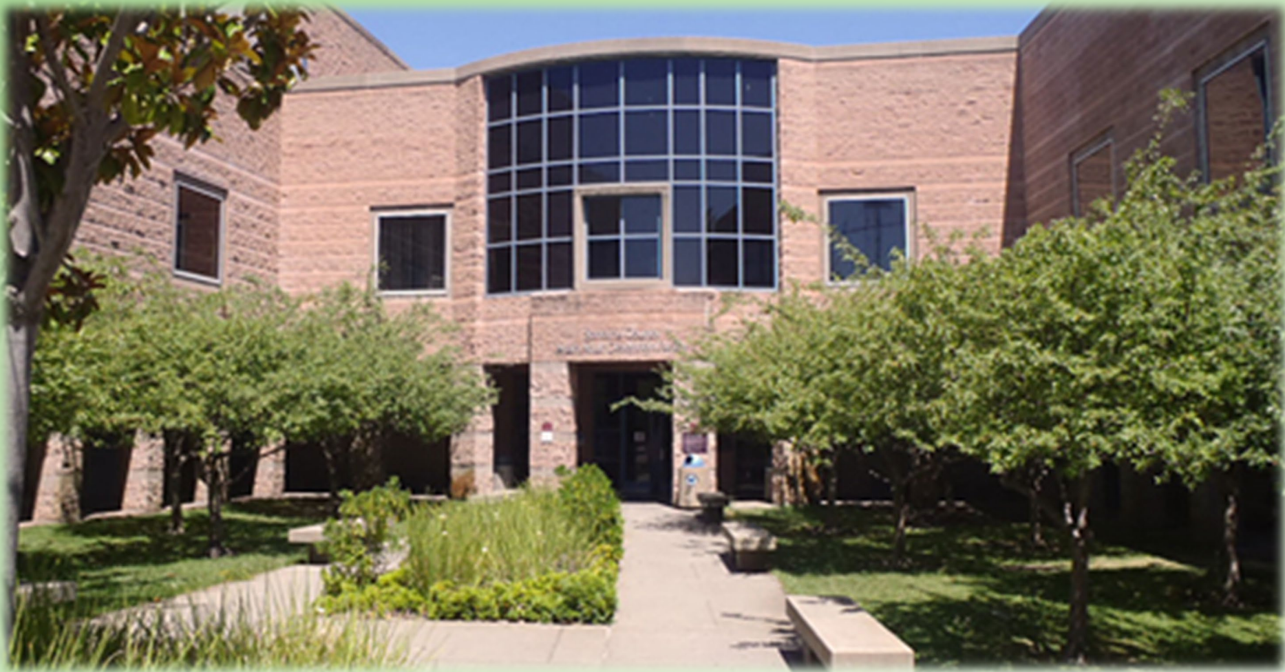
Main Adult Detention Facility
