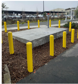
Backup Generator Poured Concrete Slab
