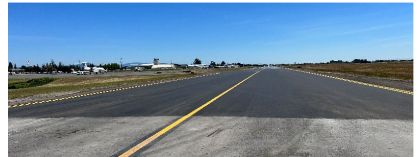
Taxiway A Rehabilitation
