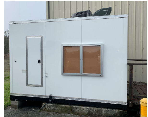
Apron F Restroom
