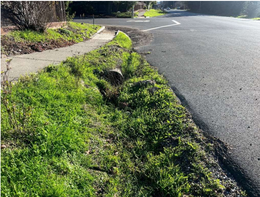
Photo 10. Photo Point 10 (PP10). Sample Point for Ordinary High Water Mark (OHWM) 1 taken in a vegetated roadside ditch adjacent to the developed pathway and Mirabel Road. Photo is oriented south.
