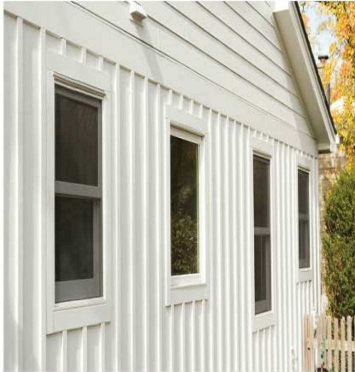
HARDIE PANEL VERTICAL SIDING BOARD AND BATTEN
