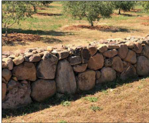
DRY STACK LOCAL STONE WALLS
