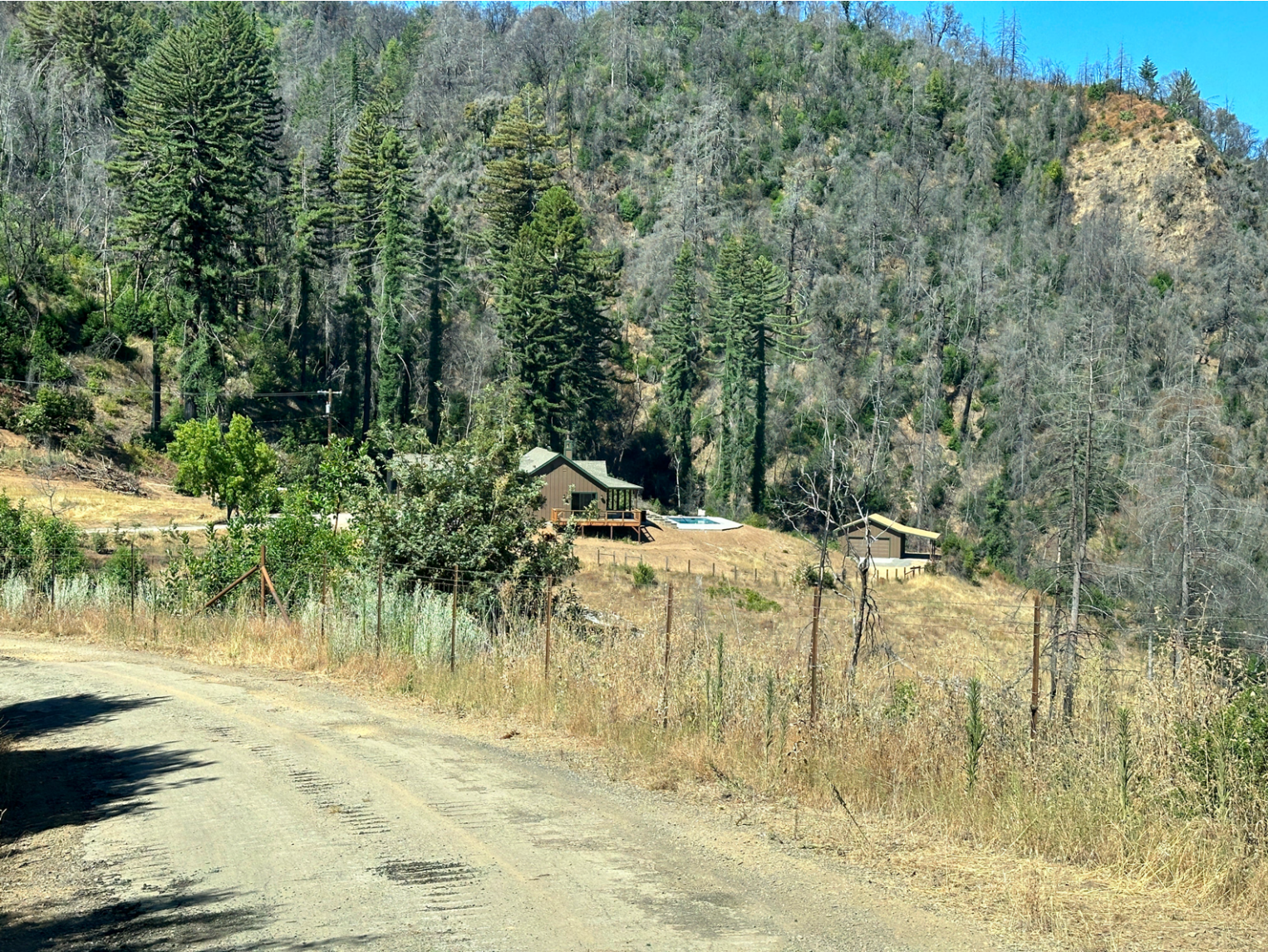
Area visible from county road; newly constructed ranch house
