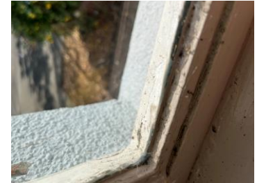
Existing first floor single-pane windows
