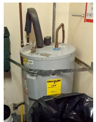
Electric resistance water heater in Janitor's Closet to be replaced
