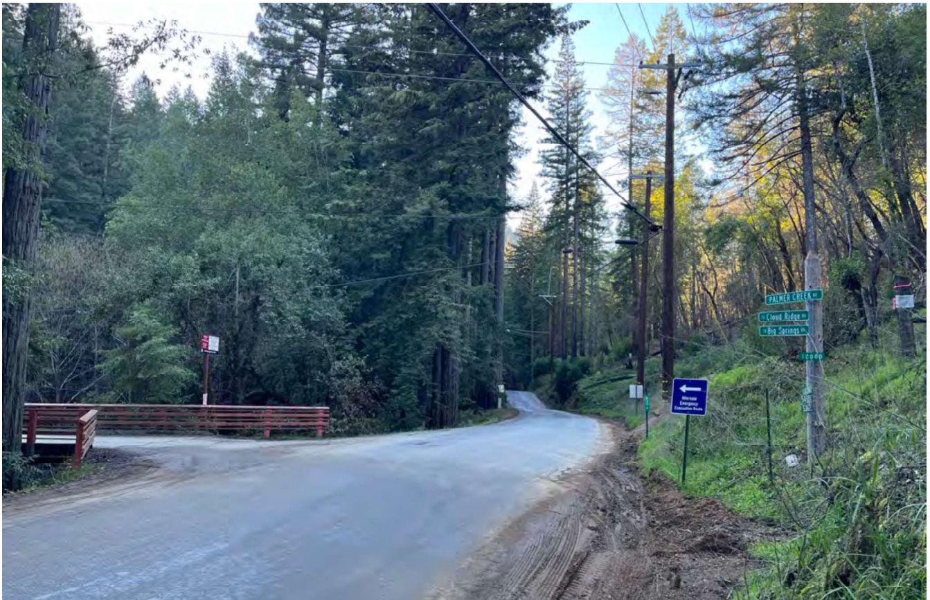
Fig 20. Sign of Alternate Emergency Evacuation Route on Mill Creek Rd. @ Palmer Creek Rd.
