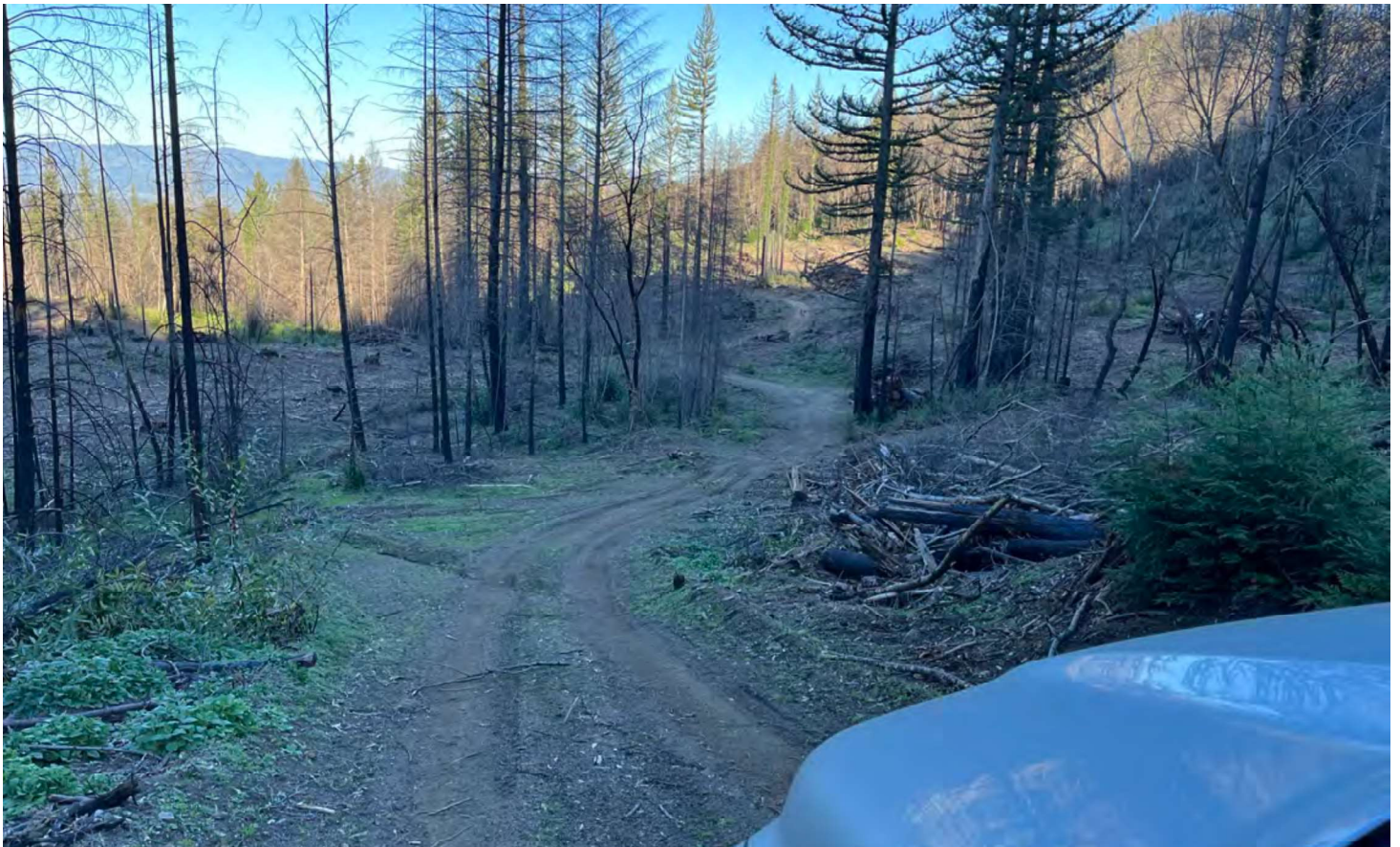
Fig 18. Adjacent Parcels Driveway looking South toward Palmer Creek Road Road
