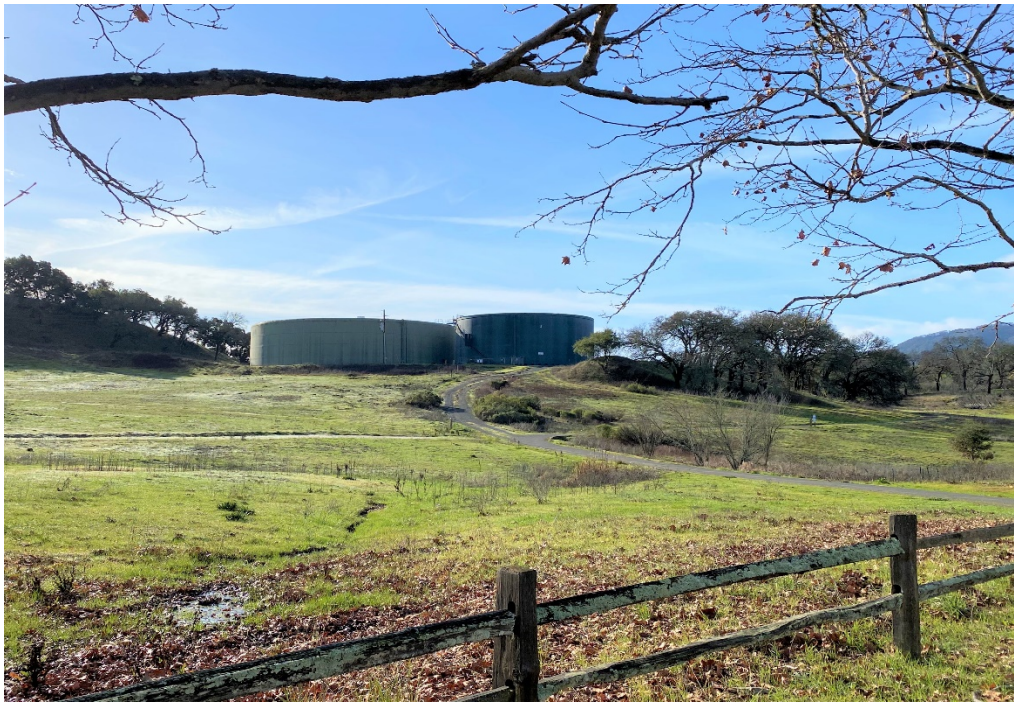
Sonoma Water “Eldridge” storage tanks at Sonoma Valley Regional Park
