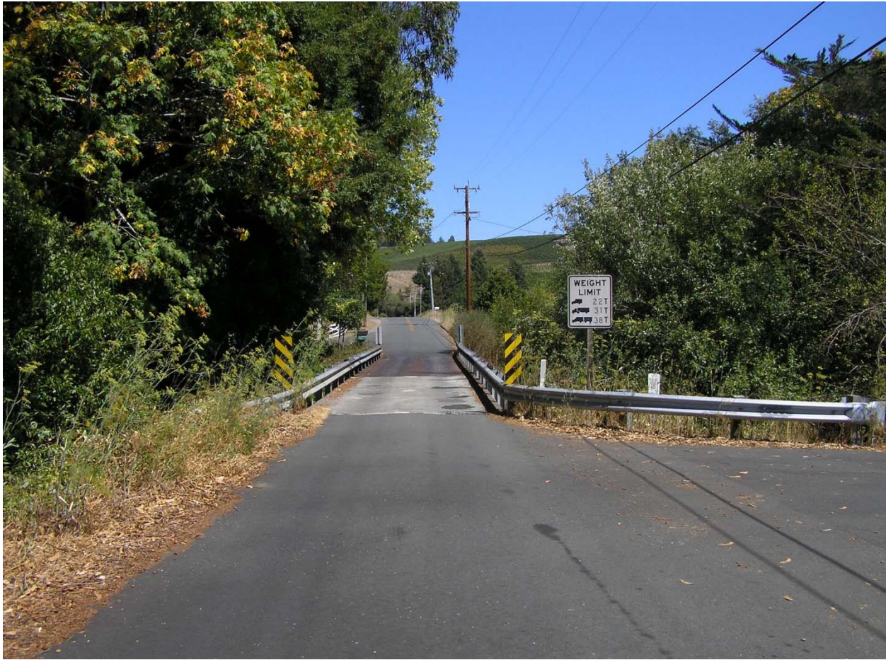
Figure 8 View of Freestone Flat Road Looking Northeast
