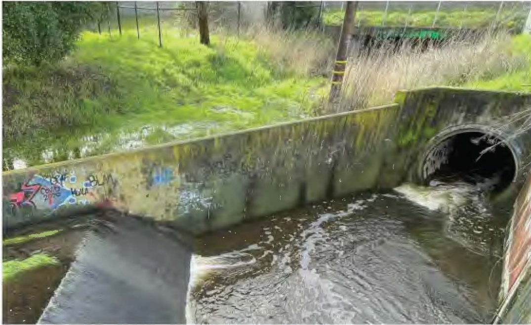
Figure 1. A representative pipe that merges with a box culvert, planned for large trash capture infrastructure project implementation. This site directly outfalls to the Petaluma River. Project will reduce trash by 9.9% the City's baseline trash volume, sourced from priority land use areas and allow for direct cleanup. This project represents five project tasks that the North Bay Water Quality Partner Project will accomplish over the next four years to help meet the requirements of the State Trash Amendments. 38.260702, -122.463629 is the representative point for our regional partnership project. Though no project is located exactly there, it is central to Petaluma, Sonoma, Sonoma County, and Napa Projects.
