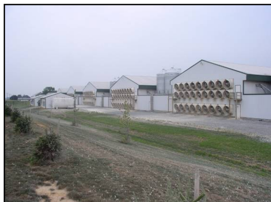
The exhaust of this multiple fan poultry house is effectively deflected by the berm and plants. Due to the quantity of fans the distance between plants and exhaust fans is much more than usual, 150 feet shown here. Irrigation is important for plants in this situation as the soil dries much more quickly due to the slope. Photo by PA NRCS.
