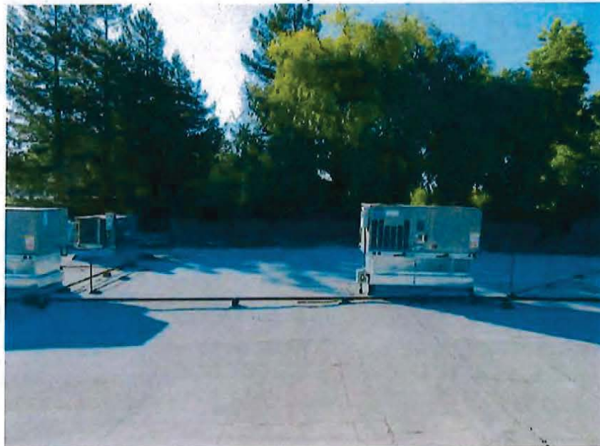
4. Roof of 2225 Challenger Way.
