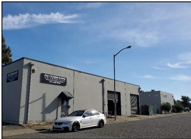
Single-storied Industrial Space
