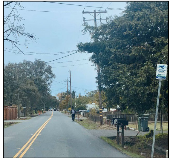
Lack of Sidewalks in Residential Area
