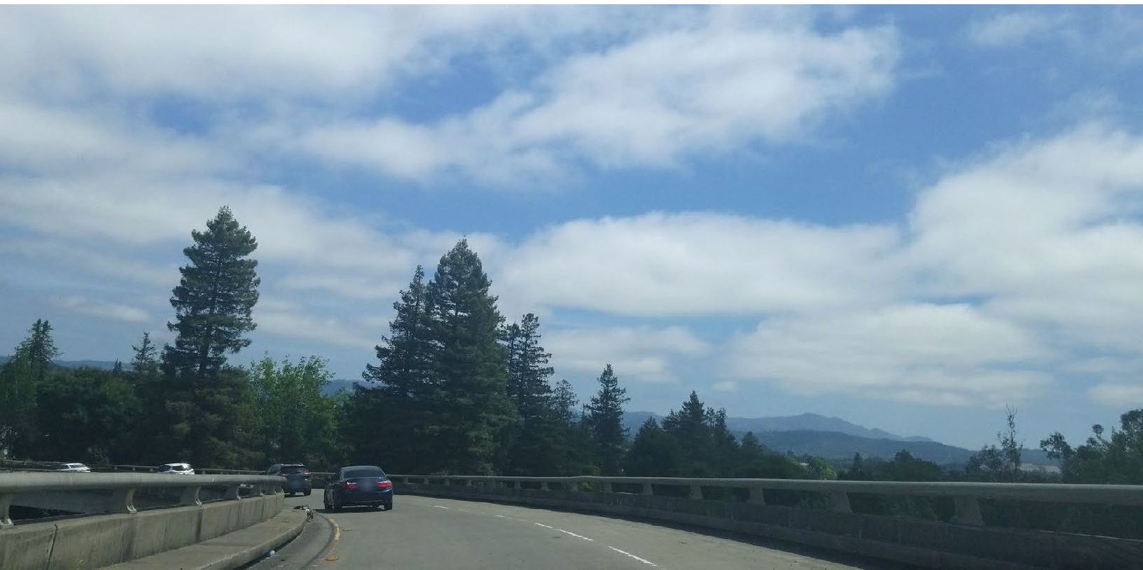
U.S. Highway 101 and State Highway 12 interchange
