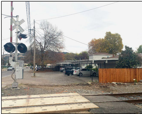
Lack of Sidewalks in a Transitional Area
