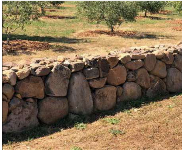
DRY STACK LOCAL STONE WALLS
