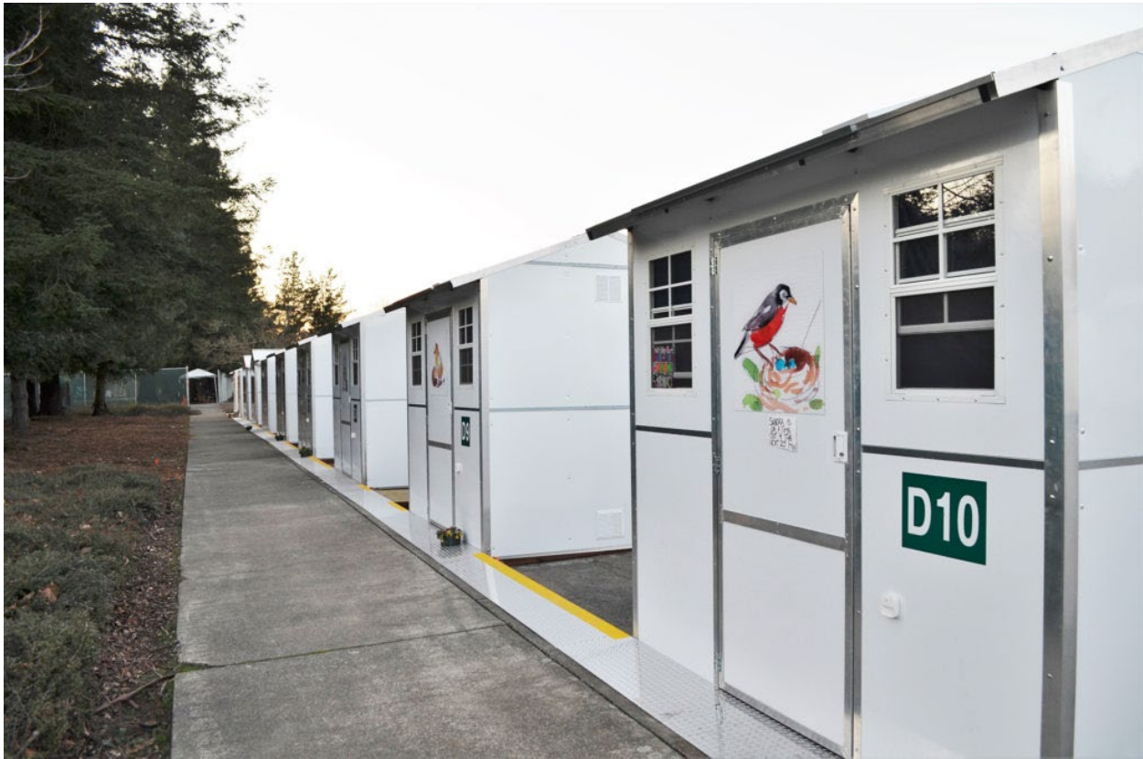
Figure 5: Los Guilicos Transitional Shelter Units
