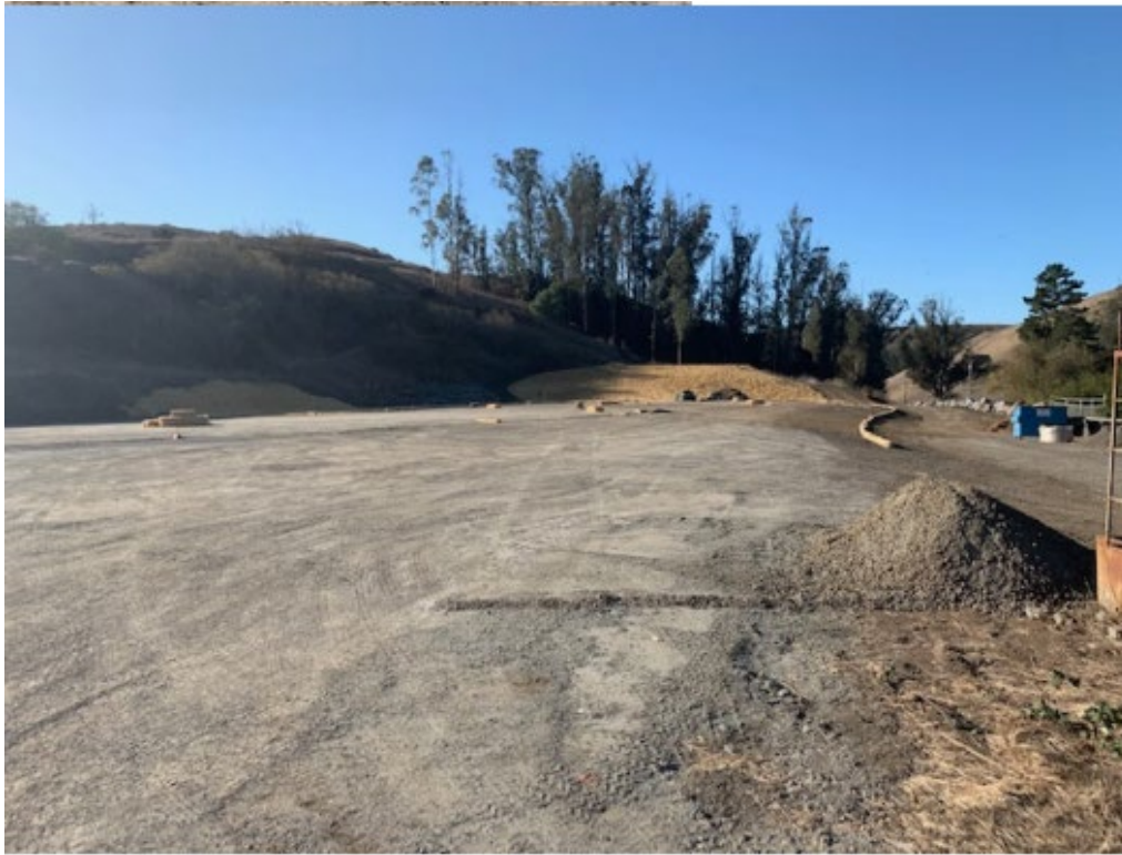
Project Site facing southwest, Bloomfield Road is to the right
