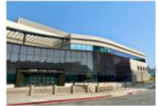
CONTRA COSTA COUNTY BUILDING
