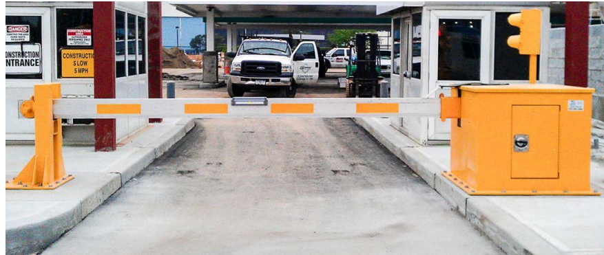
Figure 4. Crash-rated vehicle drop-arm – Ameristar M530 Barrier
