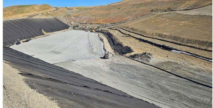
Cell R-3 Construction (April 2025)
