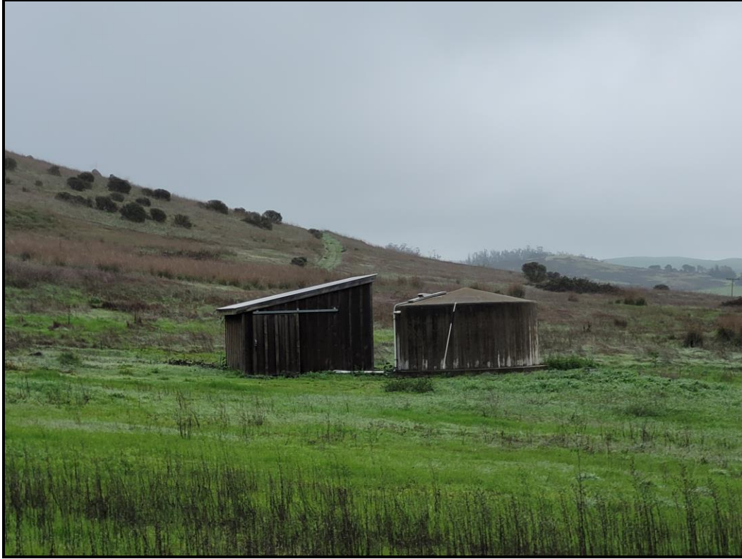
Photo 1: View of Irrigation well shed and associated concrete holding tank.
