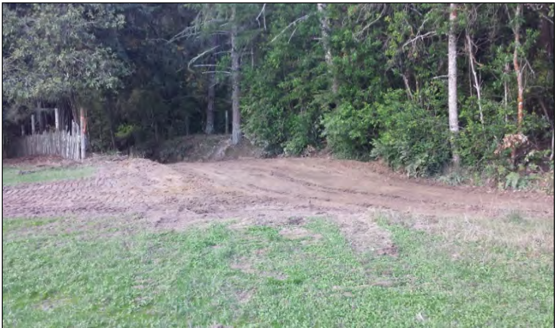
Photo 21: A properly built rolling dip used to route water off road surface.
