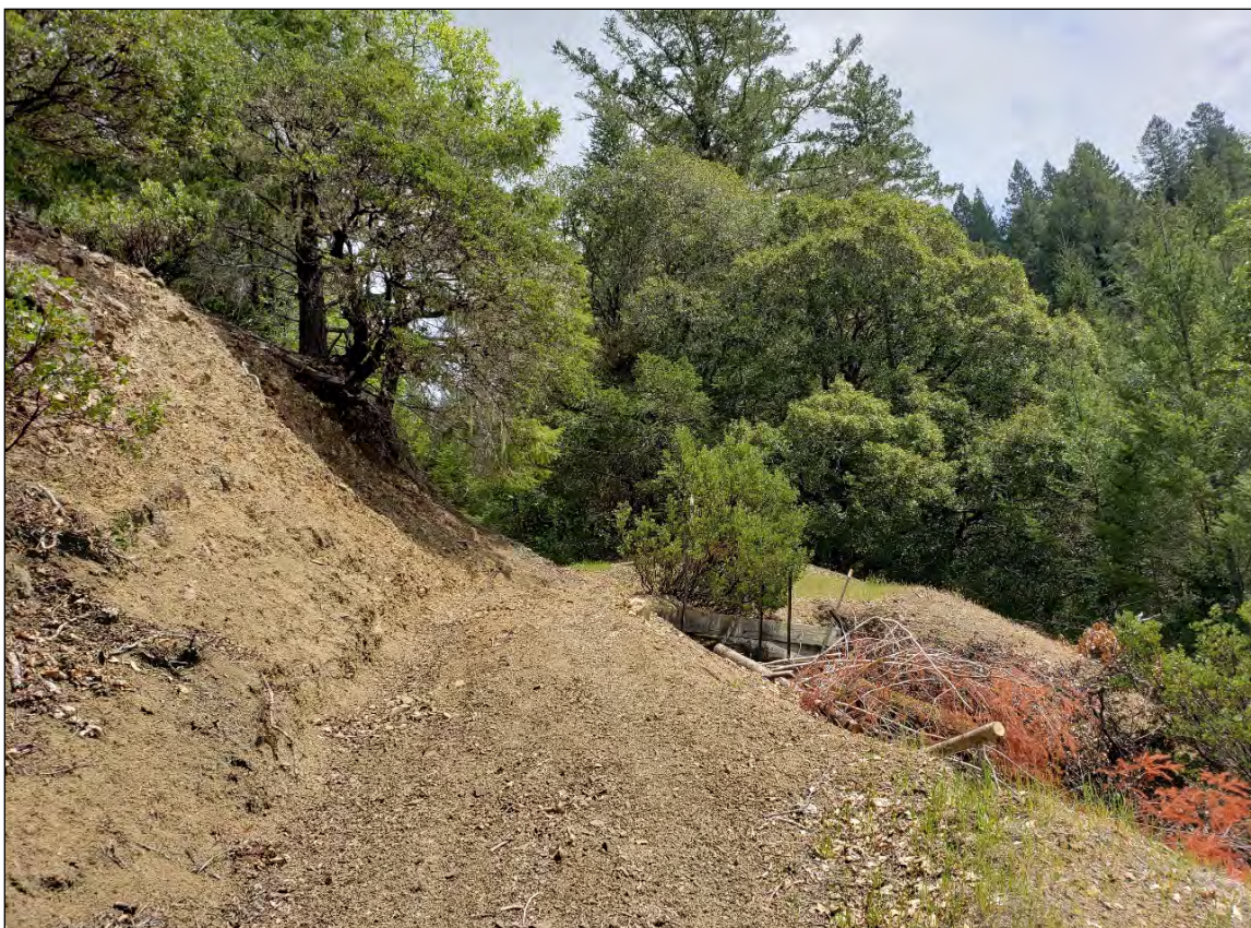
Photo 1: Poor road drainage placement (as seen on the Orange Trail) exacerbates this highly erosive landscape.
