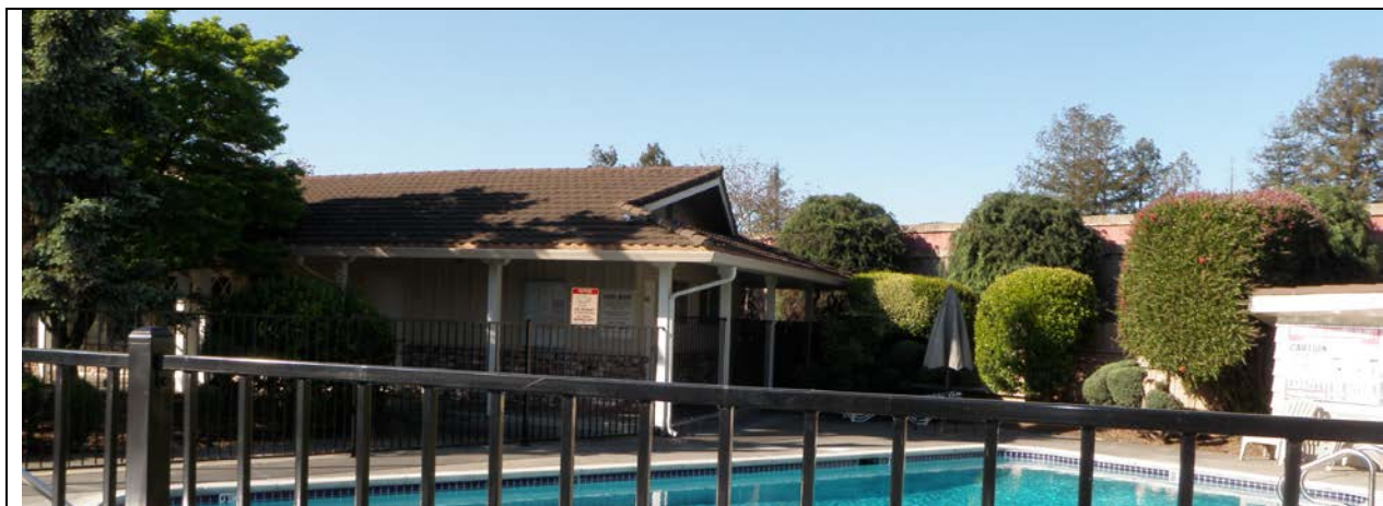
Figure 2.1.7-1: Wayside Gardens Clubhouse
