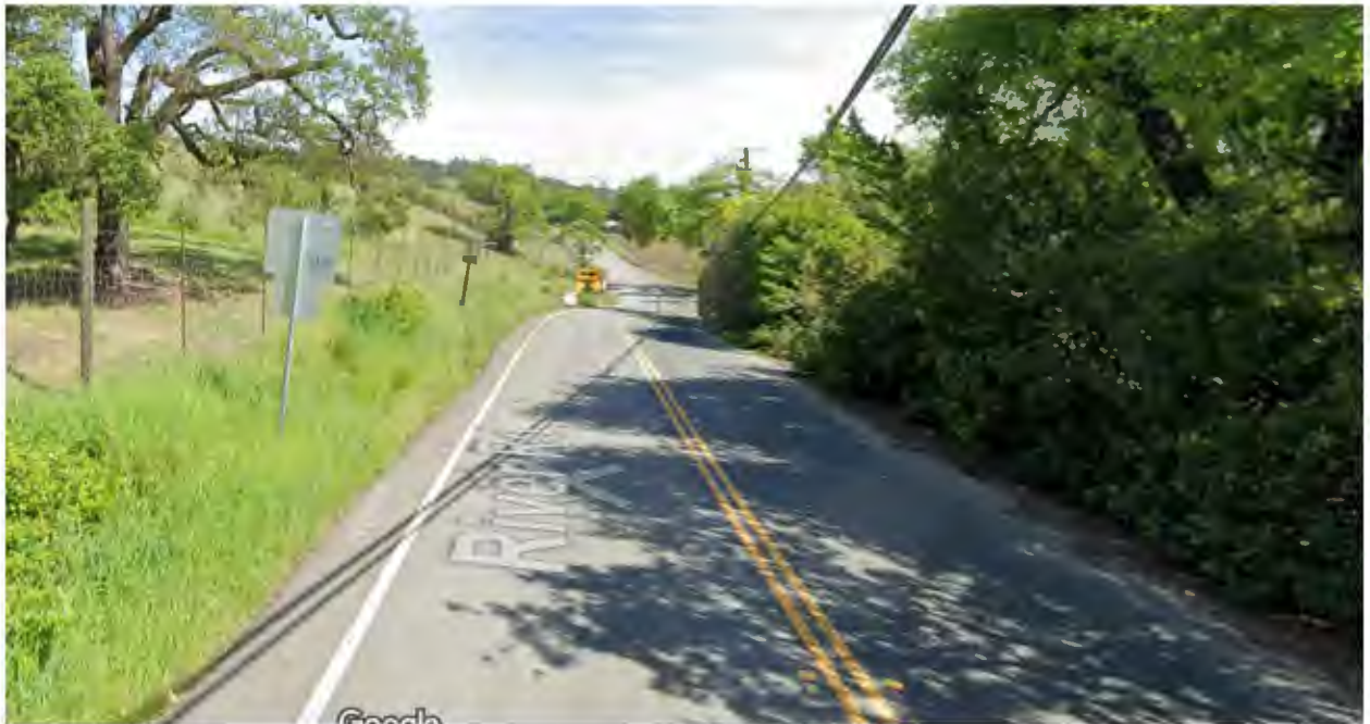
Figure 9 - Road near Washington School Road
