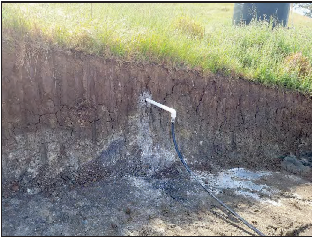
Photo 5: View of horizontal well for residence (Well #2).
