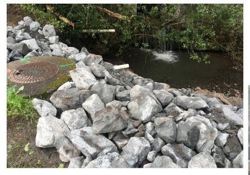
Temporary Rock was placed as an emergency, this Project will permanently secure bank and sewer infrastructure
